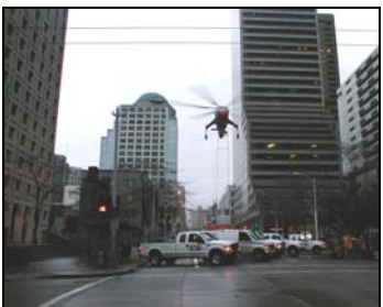
Jackson Federal Building Cooling Tower Replacement
