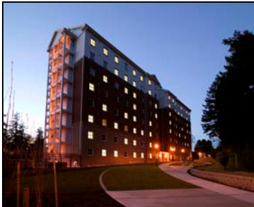
Bremerton Bachelor's Enlisted Quarters
