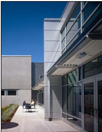
Southwest Community Center
