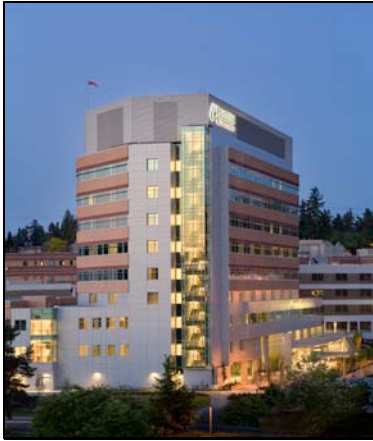
Bartlett Regional Hospital Project 2005, Juneau, AK
