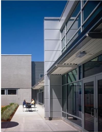
Southwest Community Center
