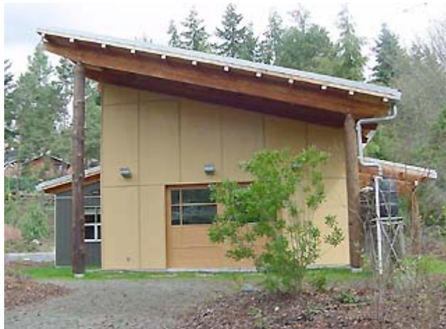
Carkeek Park Environmental Learning Center is the first city facility and the first building in Seattle registered to achieve the gold-level LEED certification. It was made from 80% recycled or salvaged construction waste, including peeler logs from a naval building in South Lake Union.
